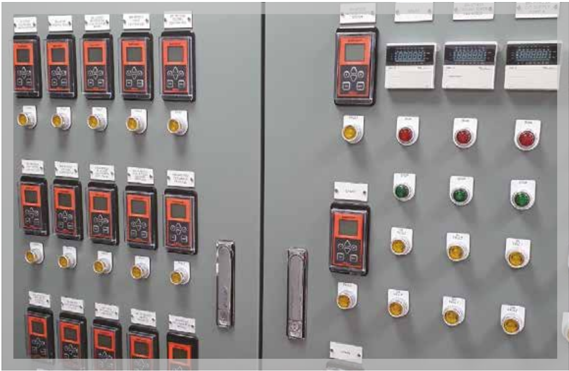
DGF-D11F (vertical type) case of ground fault relay installation switchboard
